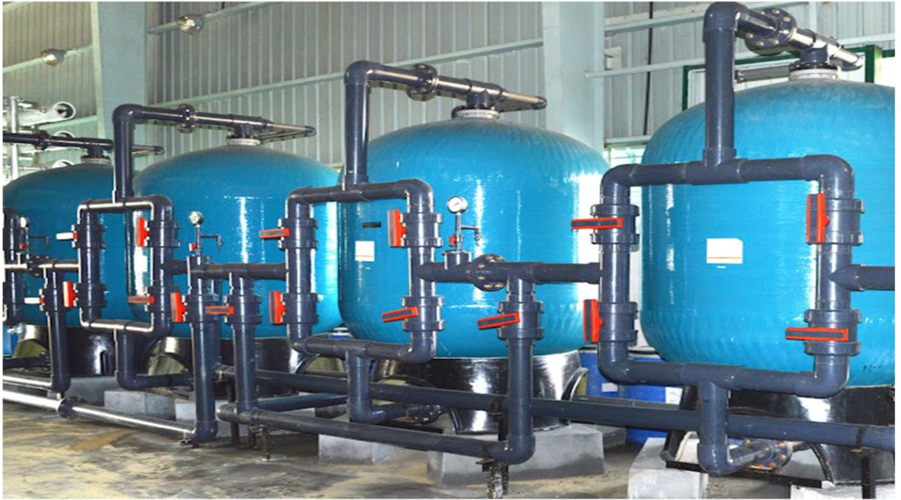
Industrial RO Plant with FRP Vessel
