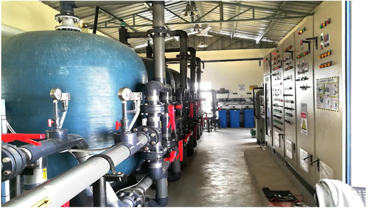
Industrial Soft Water Treatment Plant with FRP Vessel
